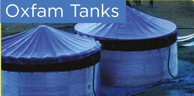
Two T95 Oxfam Tanks – Photo courtesy Oxfam
